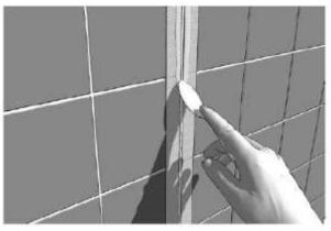
4. Finish the joint with a plastic spoon or finder tip. Wait one hour before removing tape. Remove excess silicone sealant.
