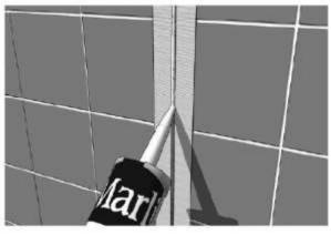
3. Apply a bead of harmonizing Silicone Sealant
